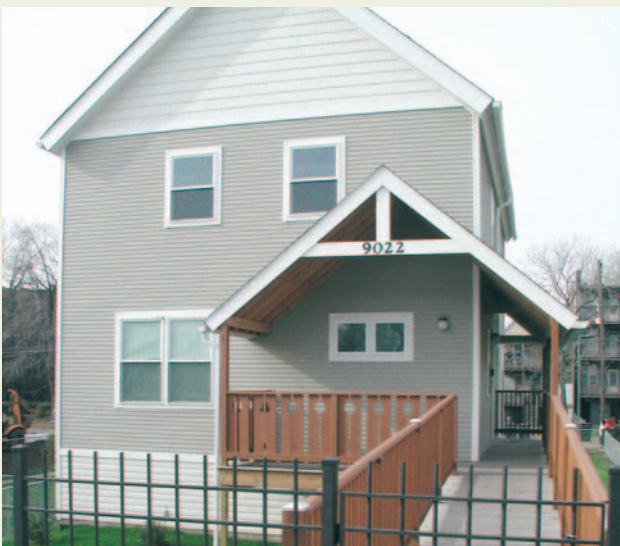
Single-family home in Chicago's South Chicago neighborhood, developed by Claretian Associates
